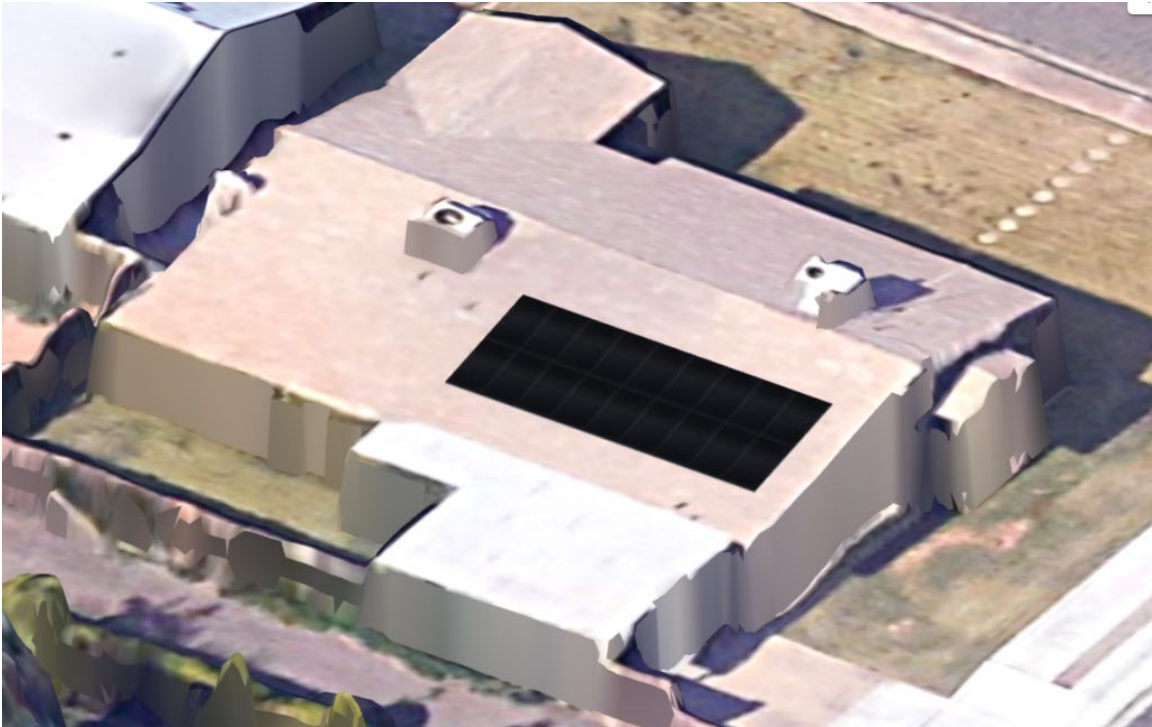
Figure 3-1: 3D model of the SW System created by PVEL in the Application.
